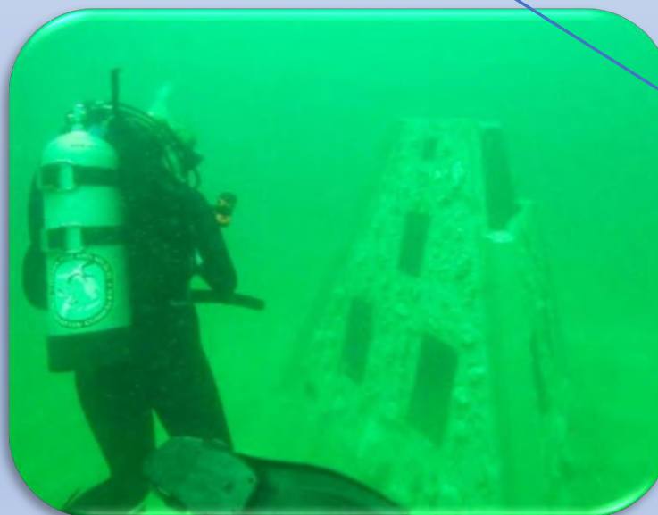
Photo 2. Diver inspects small tetrahedron, 8ft tall and 10ft base width.
