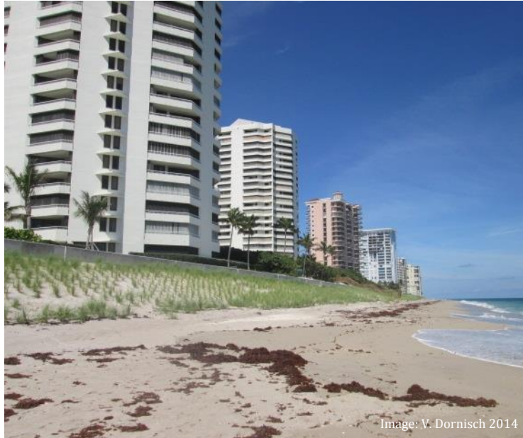
Figure 5. A newly constructed multi-building seawall, fronting the Ocean’s Edge, Condado, and Seawinds condominiums.
